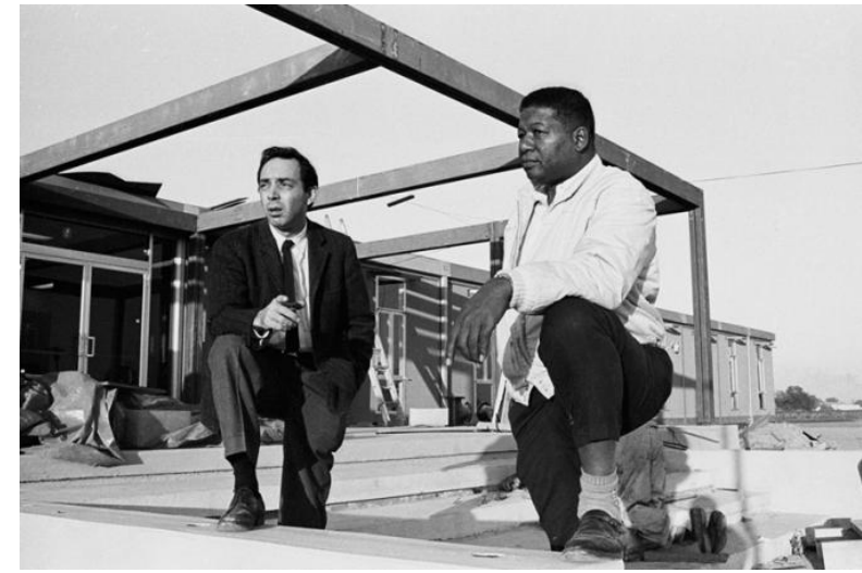
Right: Dr. Jack Geiger and Dr. John Hatch during construction of new Delta Health Center building, 1968
